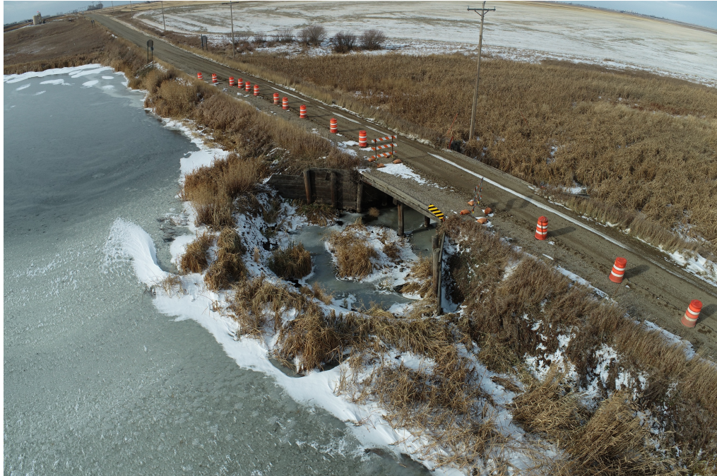
Figure 2. North Star Dam
