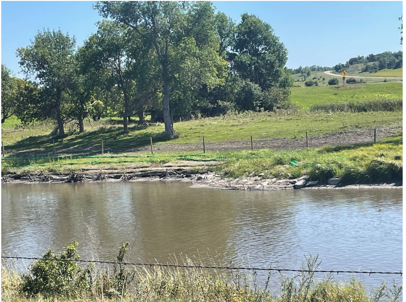
Graded bank with installed toe wood along with cattle fencing
