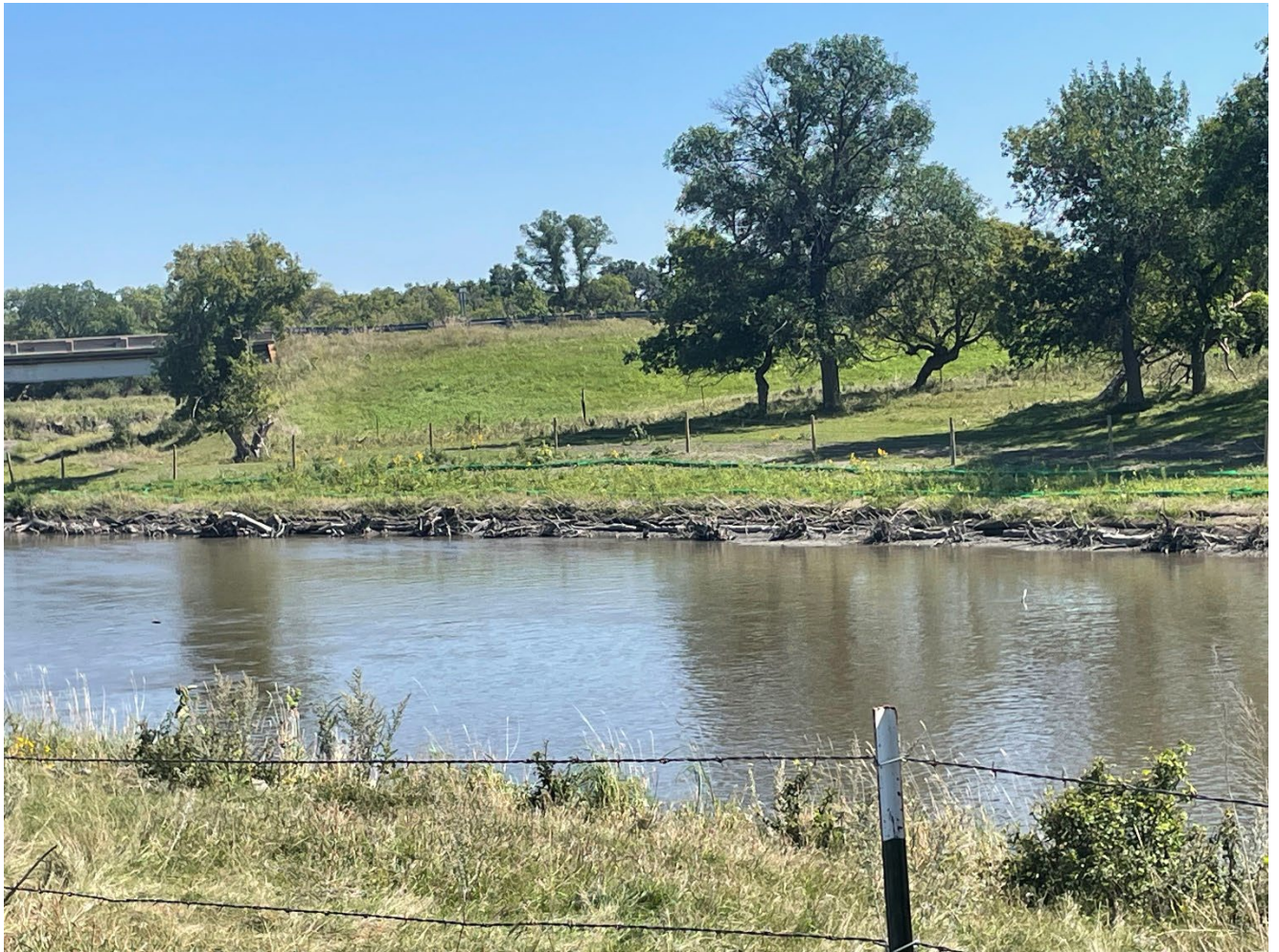
Installed tow wood with graded banks and bio logs along with cattle fencing on either side of the bank
