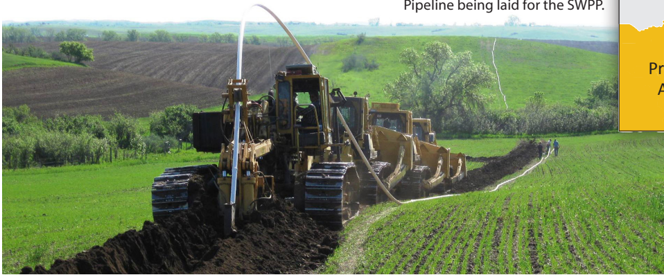
Pipeline being laid for the SWPP.
