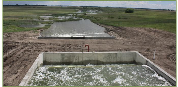
Water Commission, and is designed to prevent a potentially catastrophic overflow if the lake rises to the natural overflow elevation. Discharge through the structure is controlled by stop logs which are kept approximately one foot below the lake elevation.
