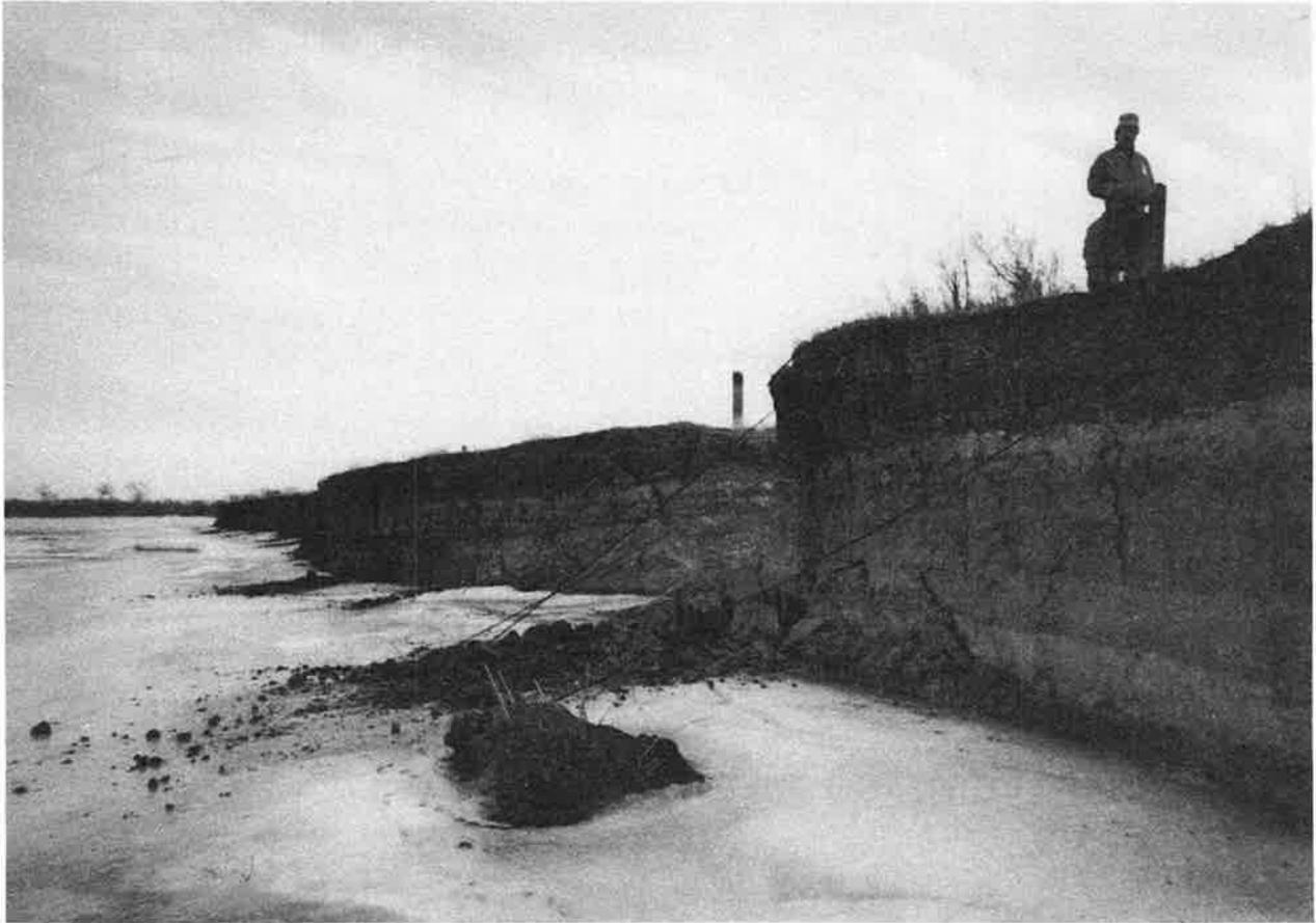
Recent mass wasting is evident as freshly fallen soils accumulate on the river ice (February, 1990). The cables are remnants of previous attempts to stabilize the banks. The landowner at this location noted that the local power company had moved power lines along this reach, and the bank recedes at an average rate of about 5 feet per year. This erosion site is about 9000 feet long.
