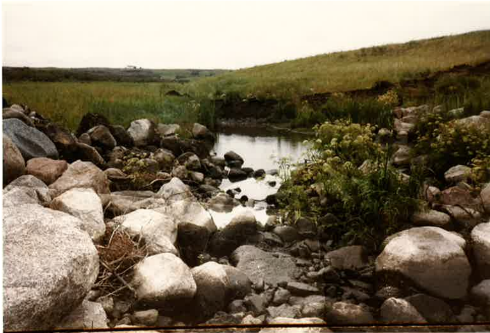
Photo No. 3 - View of downstream area and Earthen Cofferdam.
