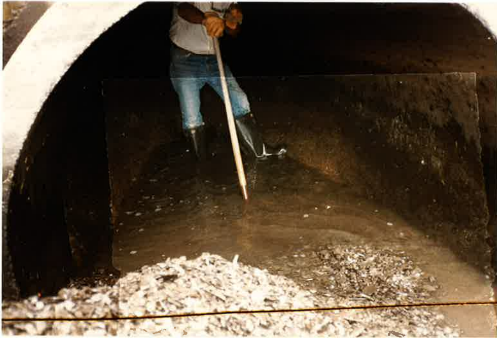
Photo No. 5 - View of Arland Grunseth inside of Conduit. To get the shale out - we had to shovel it out.
