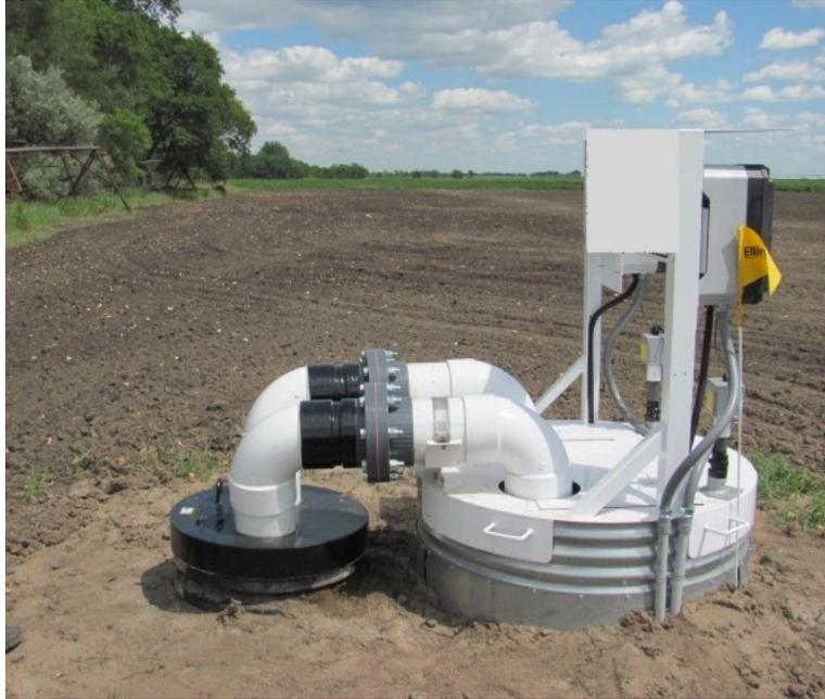
Figure. 3. Sump and lift station for the Venlo drainage project.
