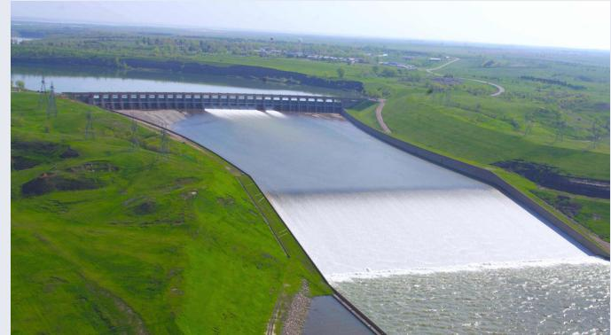
Garrison Dam was built decades ago, in part, to help control flooding on the Missouri River, the longest river in the country. In 2011, the emergency spillway gates at the dam were used for the first time to release floodwater.
