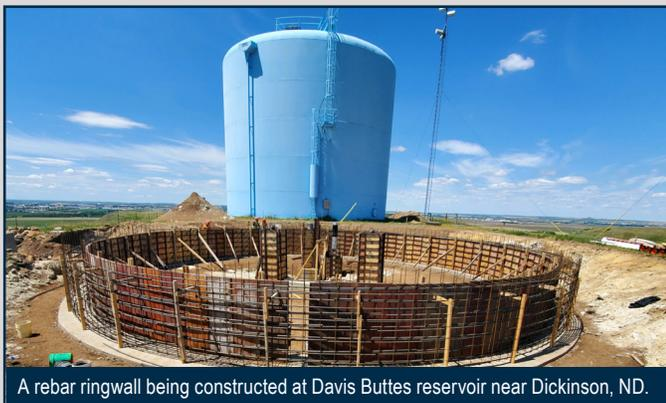
A rebar ringwall being constructed at Davis Buttes reservoir near Dickinson, ND.
