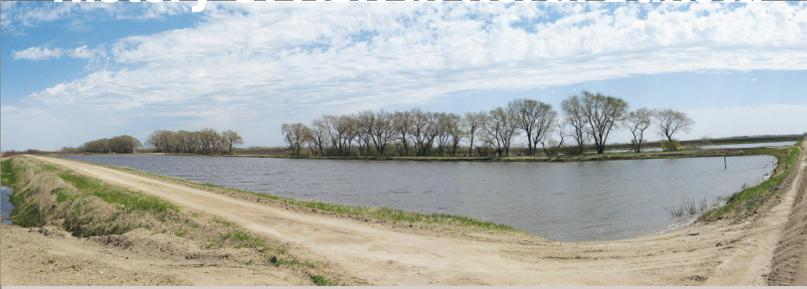
ASR project in Grand Forks County where as much as 1,000 acre-feet per year is added to the Inkster aquifer through an infiltration basin. Water is pumped from the nearby Forest River when flows are high in April to June and later extracted from the aquifer during the irrigation season.
