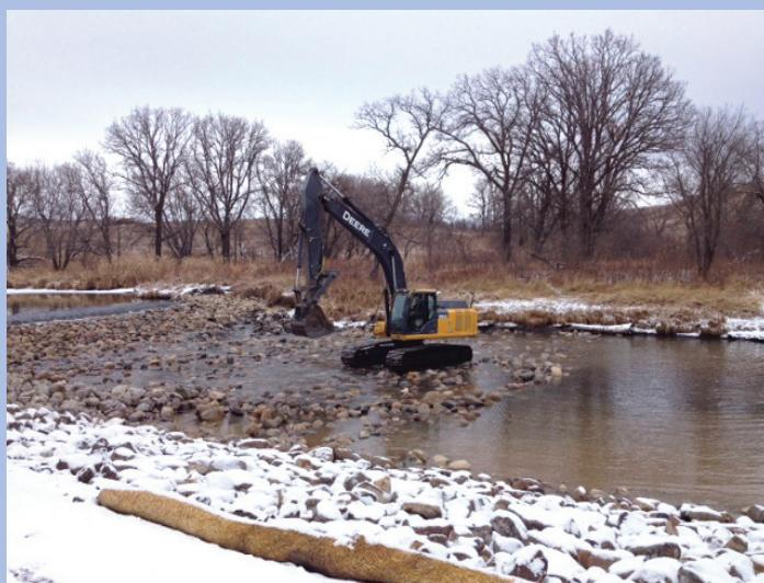
**Construction of the descending stone structure that allows fish to move upstream at Warwick Dam.**
