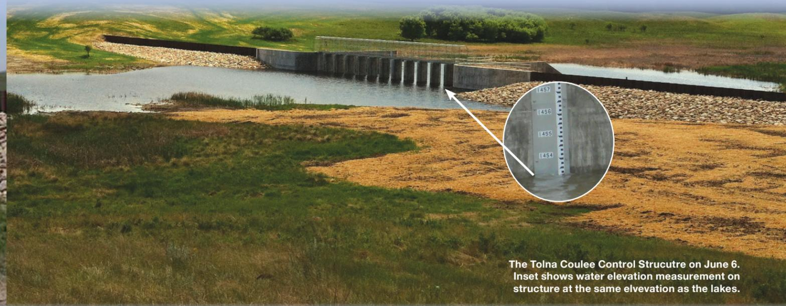
The Tolna Coulee Control Structure on June 6. Inset shows water elevation measurement on structure at the same elevation as the lakes.
