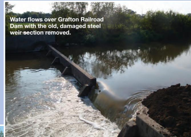
Water flows over Grafton Railroad Dam with the old, damaged steel weir section removed.
