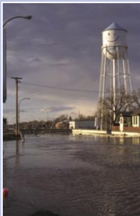
Flooding in Grand Forks, April 1997.
