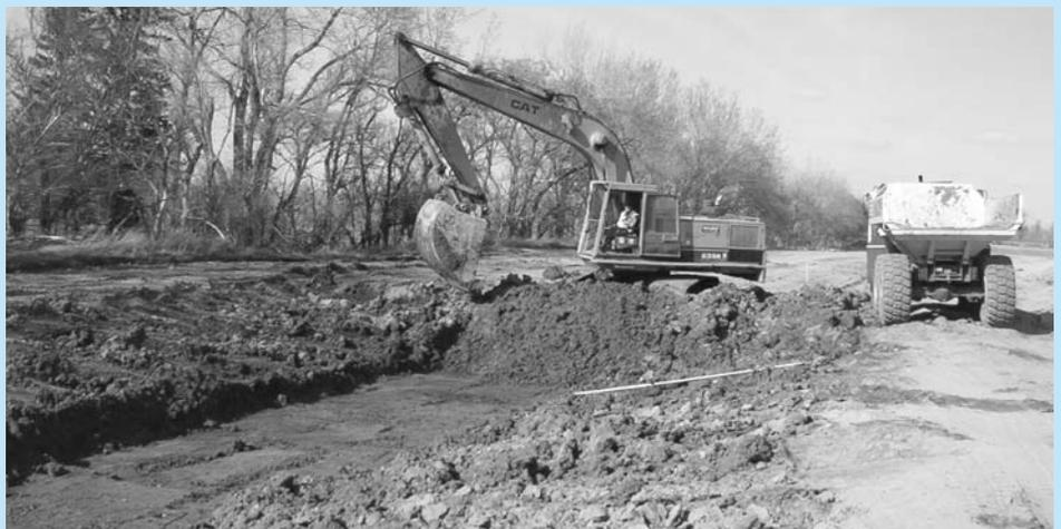
Workers are excavating the outlet channel near Long Lake. The excavated clay is being used to line other sections of the Devils Lake Outlet channel.
