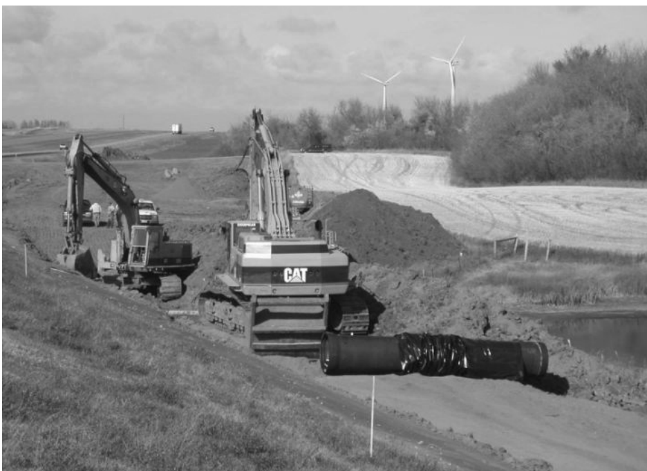
Construction on the Northwest Area Water Supply project in 2003.
