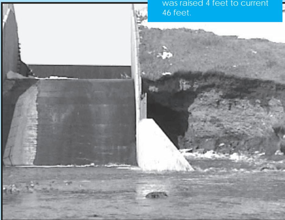
Photo 1: Uncontrolled flow occurring under the spillway of Mount Carmel Dam, March 2003.
