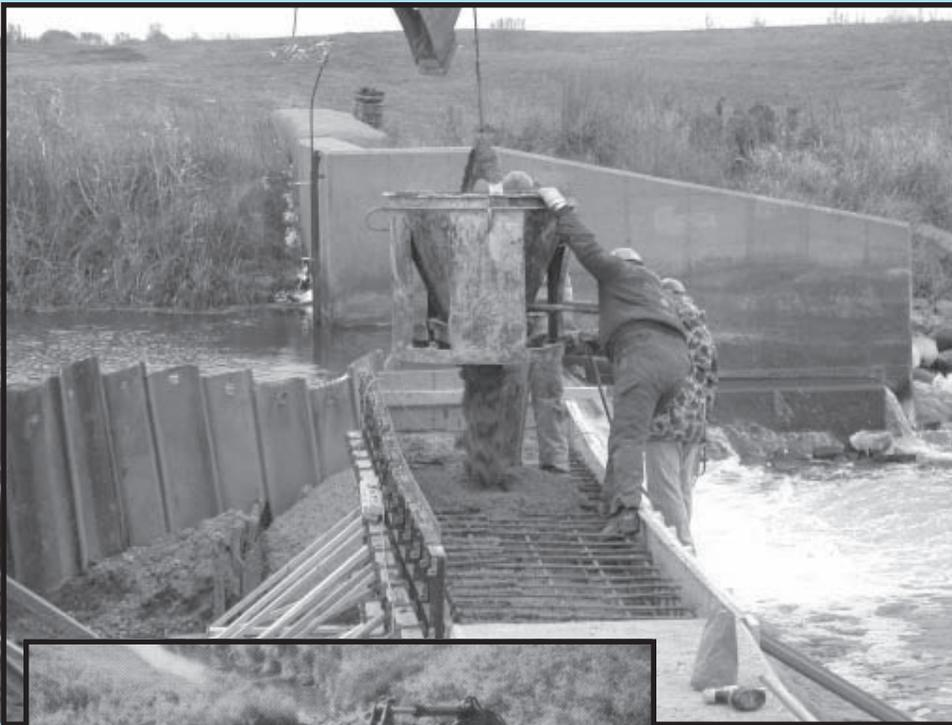
(Above) Workers are pouring a concrete cap on the existing rubble/masonry of LaMoure Dam.
