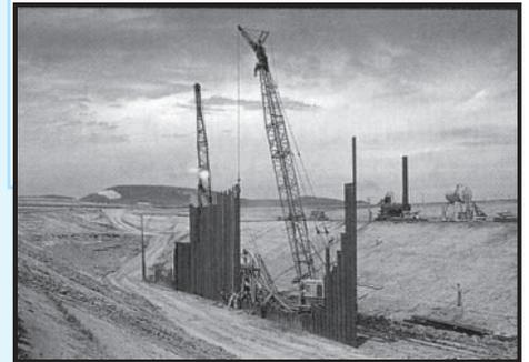
Driving sheet piling in core trench, Garrison Dam, July 1948.
