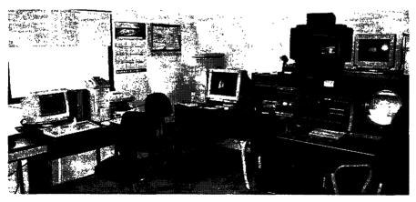
The operations area in the Stanley Radar, as it appeared at the close of the 1997-1999 biennium. From left to right are: computer for Internet access and word processing, TITAN radar data acquisition system, two-way radios and weather station display, and main radar console. Atop the console at far right is the Radar Data Acquisition System (RDAS) computer and display. (Photograph by Darin Langerud)
