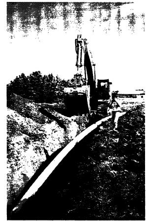
A backhoe is used to install large diameter pipe south of Hettinger in this particular phase of the Southwest Pipeline project.
