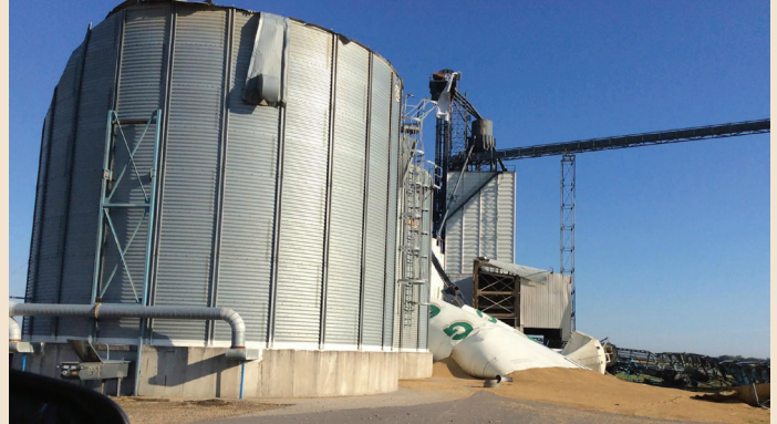
A tornado damaged the Taft elevator complex four miles north of Hillsboro on August 27, 2016. Photo courtesy of NWS Storm Survey.
