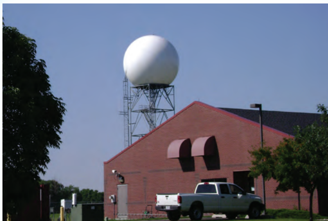
WSR-88D Doppler Weather Radar located at the National Weather Service Forecast Office in Bismarck.
