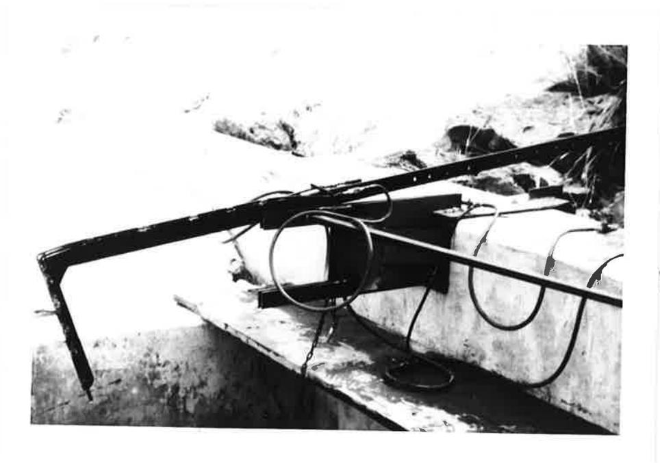
Photo 3. Pitot Tube in Stowed Position
