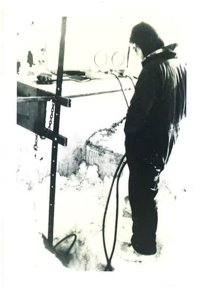
Photo 1. Pitot Tube Operating Through Ice
