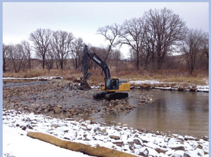
Construction of the descending stone structure that allows fish to move upstream at Warwick Dam.
