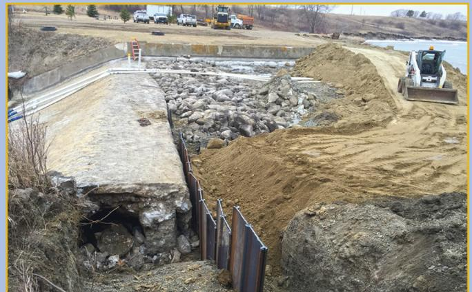
Repairs being made to Tolna Dam. The reservoir was drawn down and a cofferdam was constructed to allow access to areas needing repairs.
