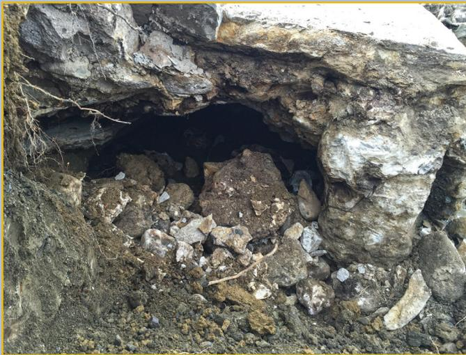
Water flowed underneath Tolna dam and caused internal erosion that can be seen here.
