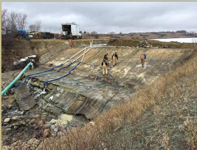
Members of the construction crew searching for voids underneath the spillway. When voids were found, grout was pumped into the structure to fill them.
