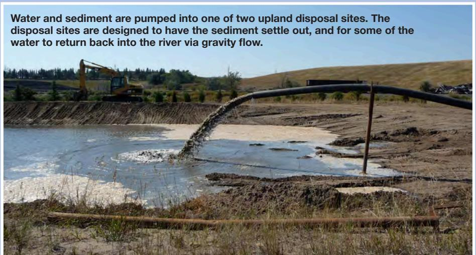
Water and sediment are pumped into one of two upland disposal sites. The disposal sites are designed to have the sediment settle out, and for some of the water to return back into the river via gravity flow.
