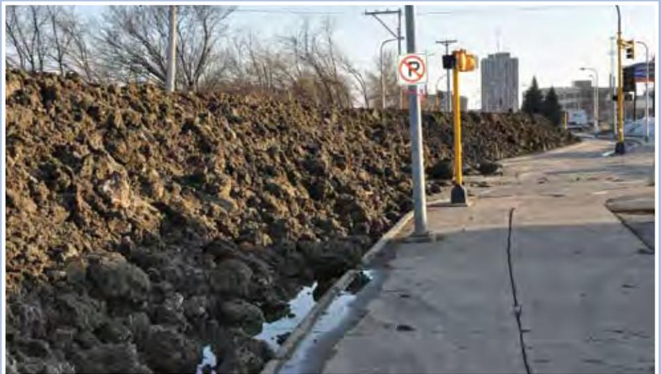
Temporary levees like this one along 2nd Street in Fargo have to be built to protect the community from major flood events like those experienced this spring. With a more permanent flood control project in place, Fargo could avoid having to build these types of structures, and avoid many of the inconveniences that occur during their construction, and after they're in place.
