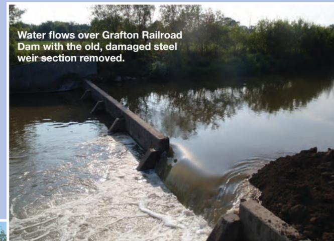
Water flows over Grafton Railroad Dam with the old, damaged steel weir section removed.
