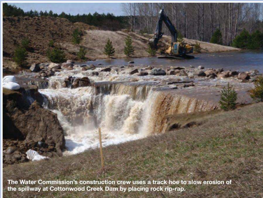
The Water Commission's construction crew uses a track hoe to slow erosion of the spillway at Cottonwood Creek Dam by placing rock rip-rap.
