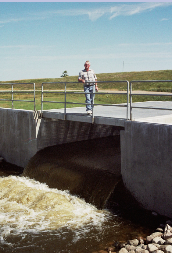
At Left: (front to back) Assistant State Engineer, Todd Sando; Jerry Backes, engineering consultant from Barlett and West/Boyle Engineers; and Bruce Engelhardt, Water Commission outlet project manager, watch as the first drops of Devils Lake water spill from the terminal structure, into the Sheyenne River.
