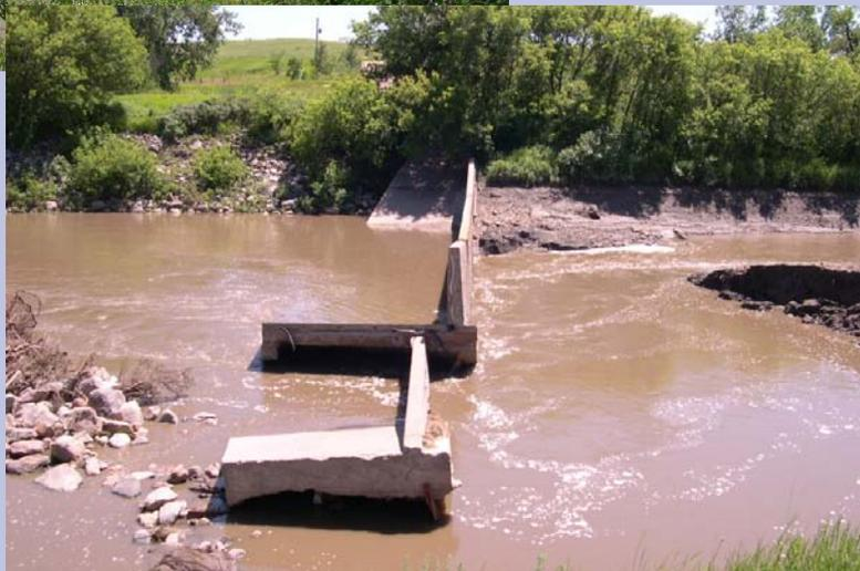
These two images show Colt Dam before its failure this past summer and after. The Water Commission's construction crew is currently in the process of removing the entire dam from the river channel.
