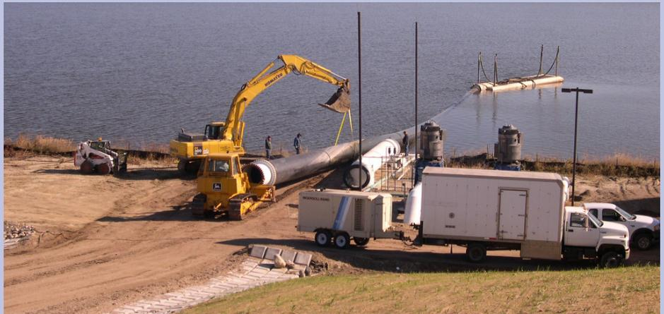
Removal of the Devils Lake Outlet Project intake pipe at the Round Lake pumping station.
