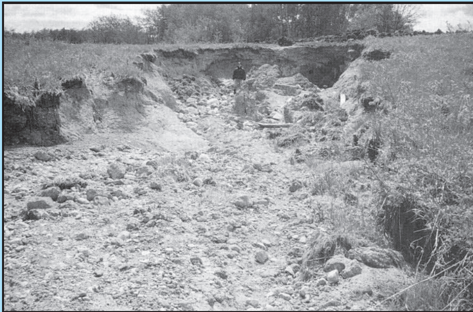
Damage caused by the overtopping of Wakopa Dam in Rolette County this past spring.
