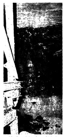
Lignite eight feet thick has to be cut through in the tunnel. The lignite separates two strata of clay, at the Garrison dam. Later programs include the mapping in  $7\frac{1}{2}$  minute units of the Pingree and Jamestown 30 minute quadrangles. The Jamestown Reservoir portion of these quadrangles will be mapped during the current field season.
