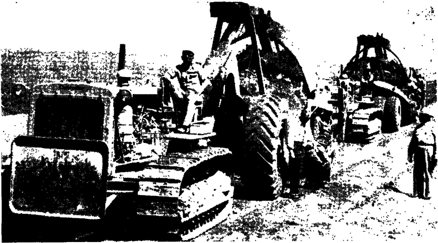
Immense machines move millions of yards of dirt
