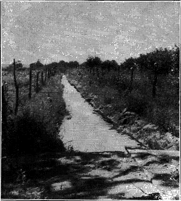
DOWN DITCHES LIKE THIS goes the water which has changed some land in Western North Dakota from a desert to fertile fields.
