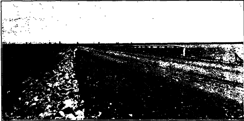
F. A. P. No. 155—Ramsey County Earth Grade with Gravel Surface near Devils Lake
